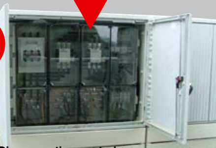
Disconnection, metering, over-current protection device
