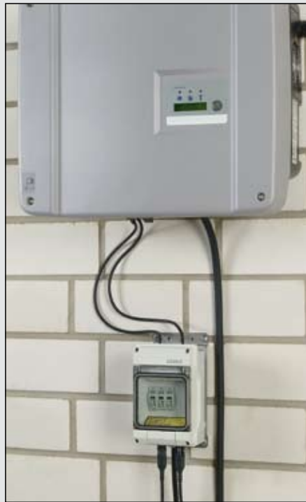
Connection to solar inverter only with DC surge arrester
